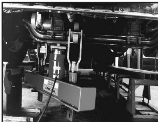
Increasing caster on right side outside of spring seats.
