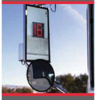
Truck loading dock distance sensing system reduces dock damage and truck / trailer repairs.
