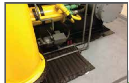
Generator Room Mat
