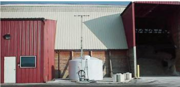
GVM's Pedestal Pre-Wet Systems are multi-function liquid deicer dispensing systems designed to pre-wet truck loads of solid de-icing materials.
