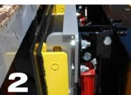
Align mounting hooks over connection bars and lower in place
